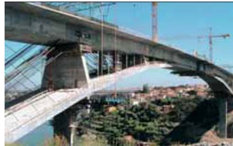
Side view of the Infant Henrique Bridge, whose arch similarly varies in width from the base to the top. The Infant Henrique Bridge has a main arch span of 280 m, while the proposed arches will have a similar proportion, but a maximum span of 250 m.
