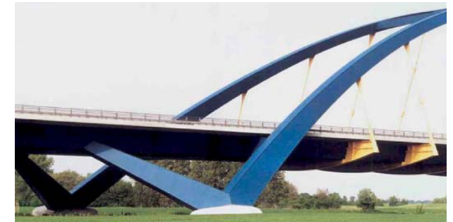
View of the angled pier and arch connection at the Bridge across the River Saale. The pier and arch form a connected structural member which brings upward force from the ground to the roadway.
